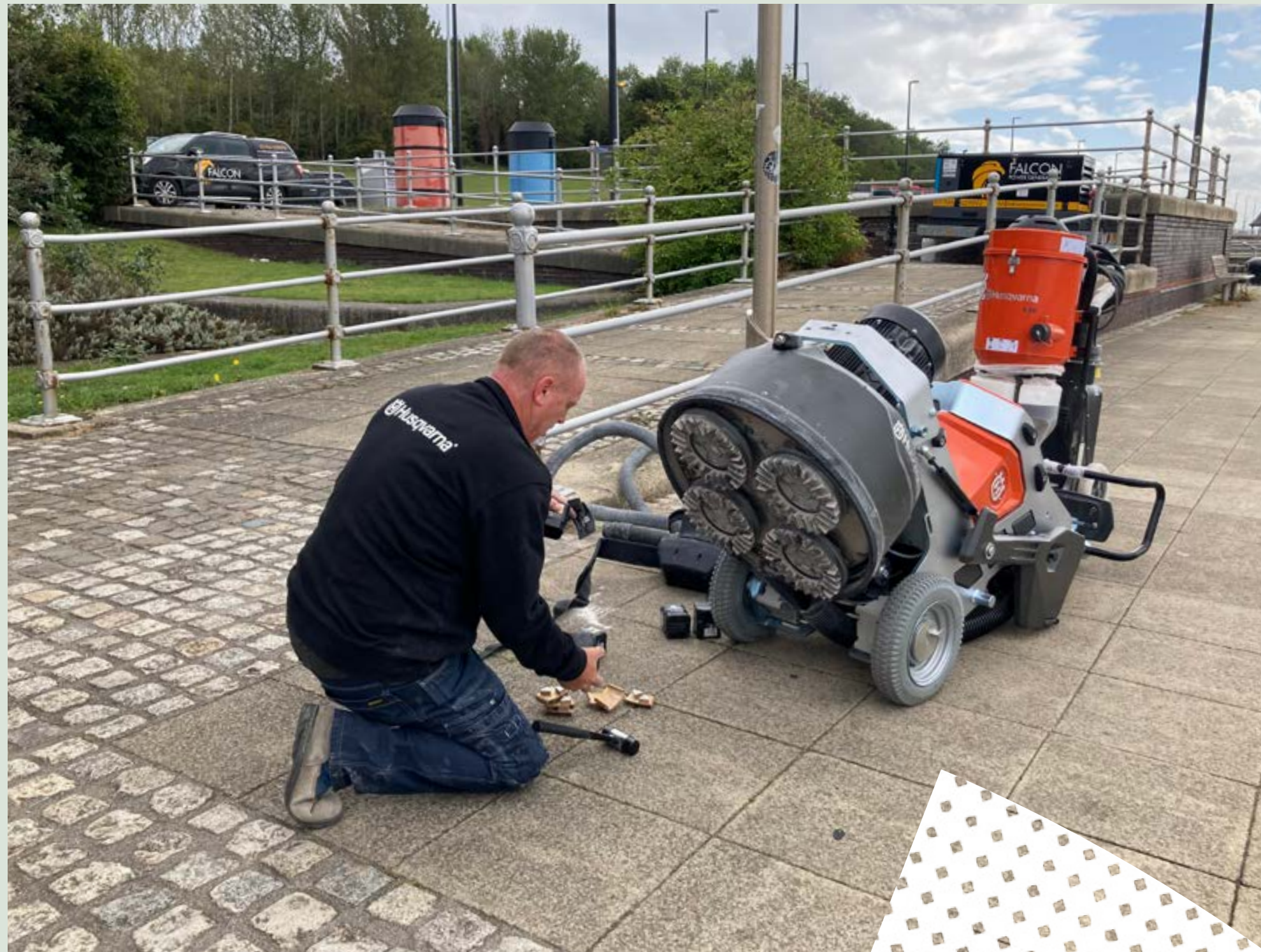
The Otterspool Promenade: Grinding granite setts to make the promenade more inclusive and accessible without the need to replace existing paving. Liverpool 2022 © Elaine Cresswell
