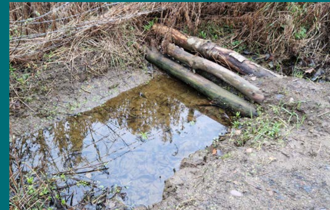
Nature based solutions help reduce the impact of climate change - newly created leaky dam in Grasmoor Country Park, Chesterfield, 2022 © Claire Thirlwall
